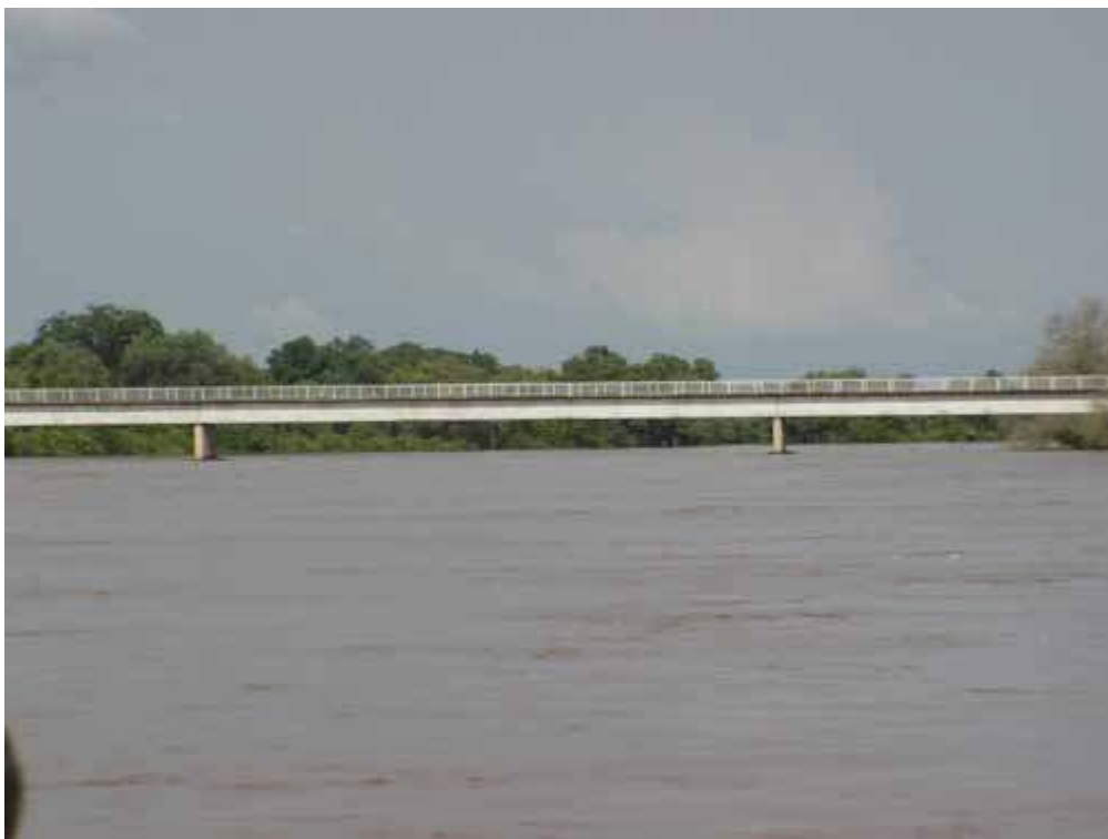
The Luangwa Bridge (water level 2ms from bridge base)
